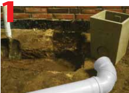
1 Dig hole to fit PointDrain and necessary pipe-work.
