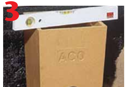
3 Position PointDrain on a 4" thick concrete slurry bed and ensure it is level.
