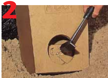
2 Drill out/cutout holes for pipe connection.
